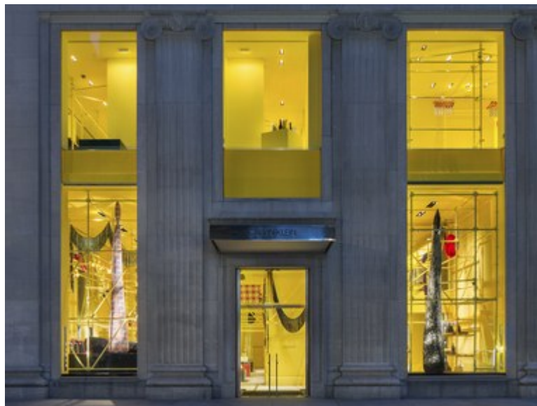
Calvin Klein's flagship Madison Avenue store has been revamped by Raf Simons and Sterling Ruby. Photo: Courtesy of Calvin Klein
